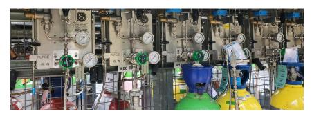
A major British chemical company uses various specialty gases to perform research and development functions. Many of these gases can pose a significant risk to workers if they are not safely contained, making leak-tight gas distribution and handling throughout more than 200 gas lines a top priority. The company took advantage of the Swagelok gas distribution program to enhance the safety of its system and realize new efficiencies.
